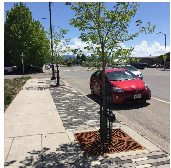
Figure 3: Completed phase 1 permeable paver system.
