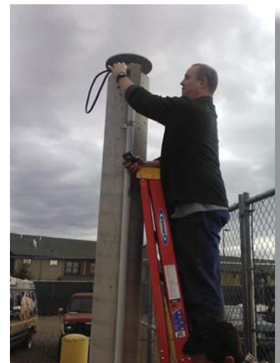
Advanced GPS mapping student Kevin Loberg installing the new base station antenna.
