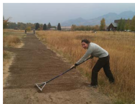
Students carried gravel in wheelbarrows to a trail near the East Gallatin Recreation area. Where they, like Heidi Clark here, then raked it out to a nice thick gravel surface that should last for at least 10 years.
